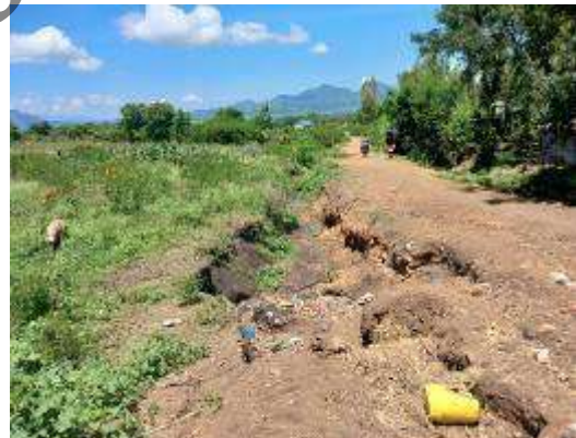
Drainage situation of area.
