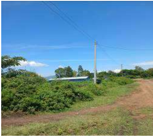
National Grid Energy access within Sofia
