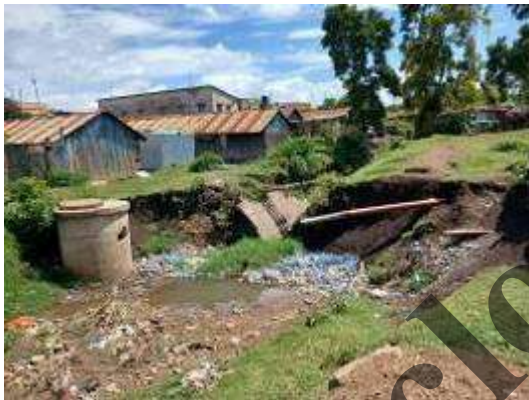
Solid waste dumped in the area
