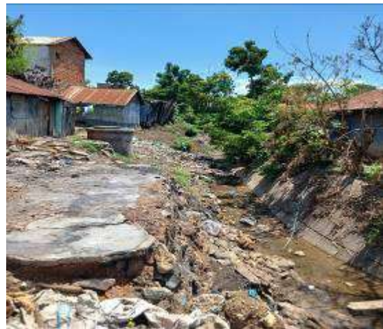
Drainage channel in the area
