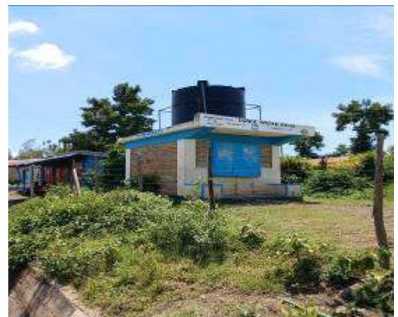
County Government water kiosk
