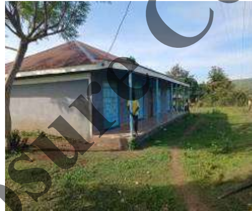
Sample housing unit in Nyandiwa.
