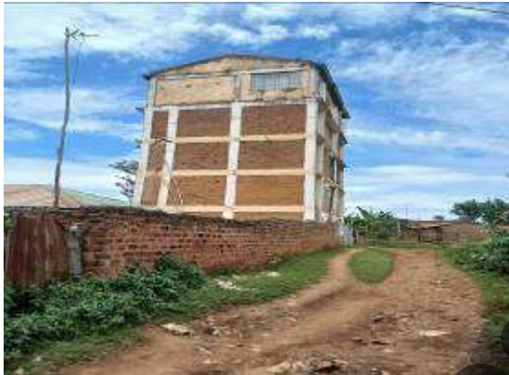
Sample Housing Structure within 1000 Street
